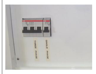
01. The three phase and single phase circuit breakers are located in the electrical module front panel behind the circuit breaker door.
