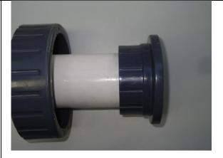
04. Using high pressure PVC solvent cement glue the valve union to the 3" (80mm) pipe. Ensure all gluing surfaces are primed with PVC solvent primer. With the unions in place tighten the collars. If required apply a suitable lubricant to the o-rings. Assembled the sheetmetal valve covers and end covers back in place.
