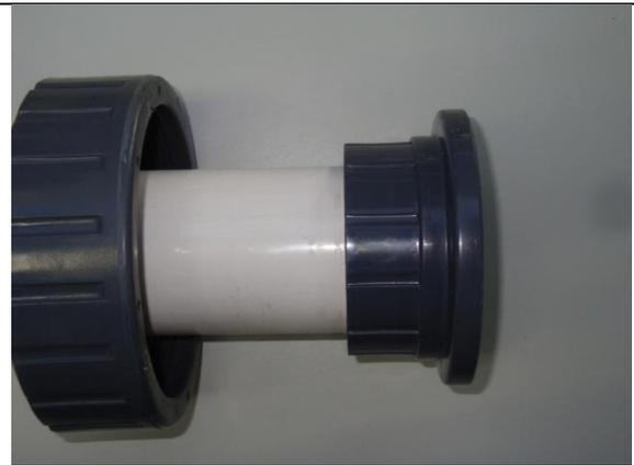
04. Using high pressure PVC solvent cement glue the valve union to the 3" (80mm) pipe. Ensure all gluing surfaces are primed with PVC solvent primer. With the unions in place tighten the collars. If required apply a suitable lubricant to the o-rings. Assemble the sheetmetal valve covers and end covers back in place.
