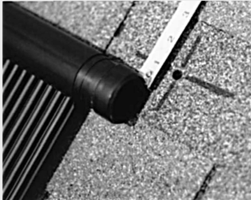
FIGURE 3 Outlet Header Bracket Location
