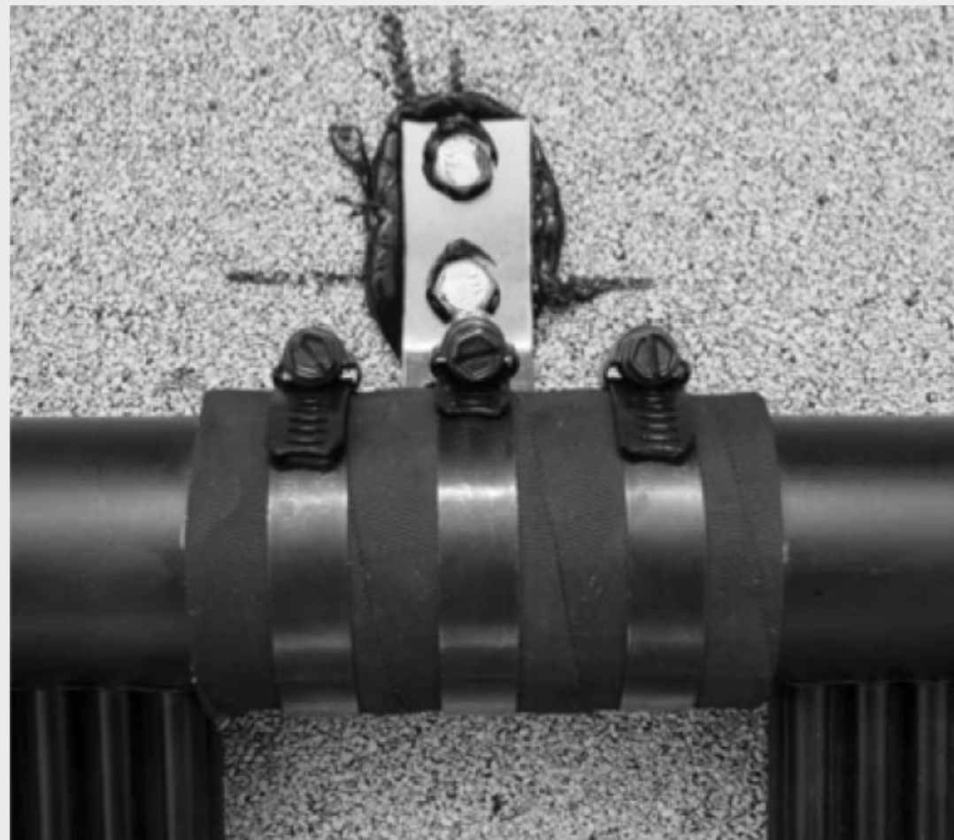
FIGURE 5 Installed Outlet Header Bracket with Hose
