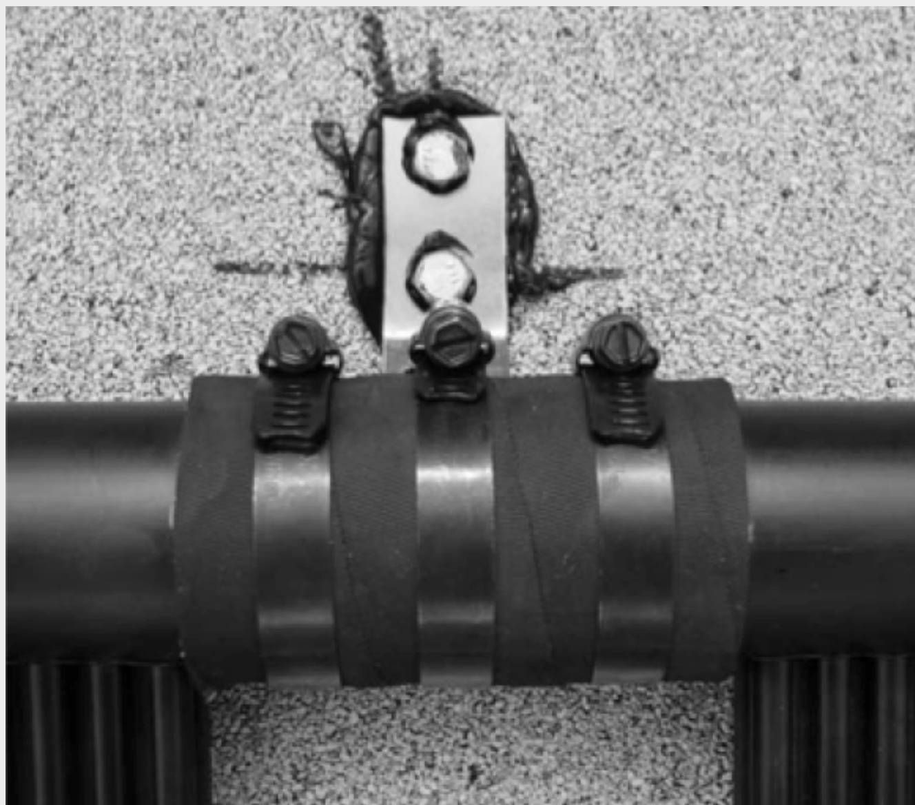
FIGURE 5 Installed Outlet Header Bracket with Hose
