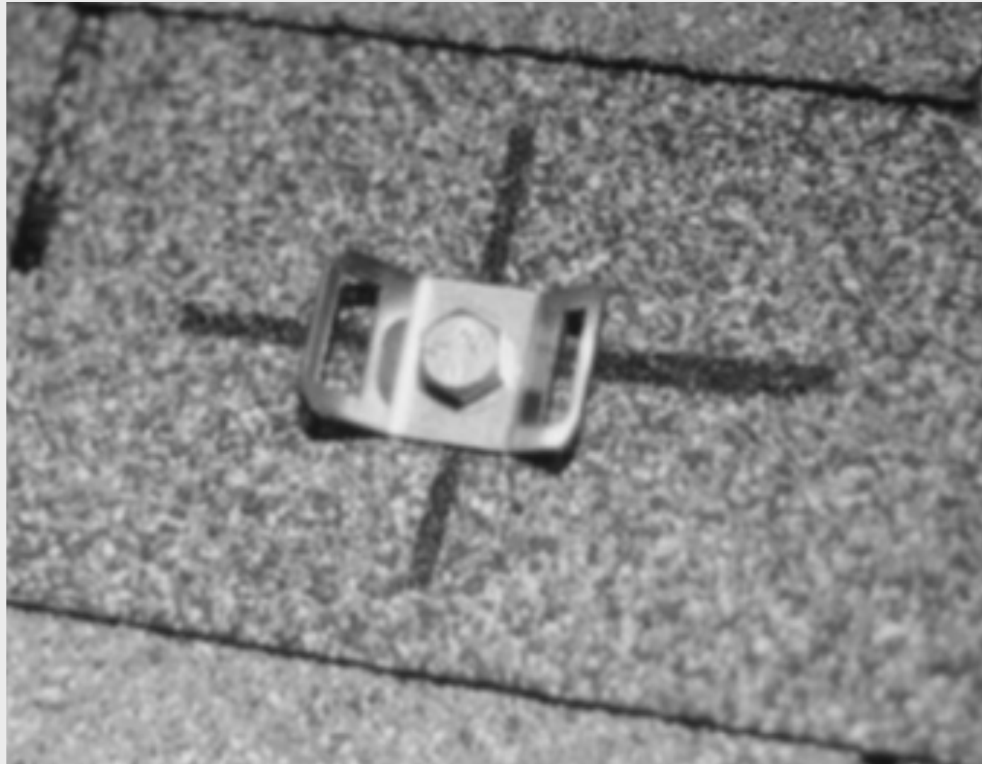
FIGURE 6 Hold-Down Strap Bracket
