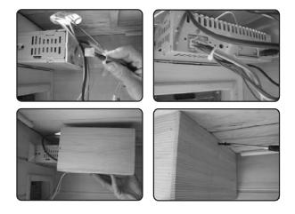
Plug the 6 pin's plug onto the 6 pin's socket of the control panel. Plug the 4 pin's plug onto the 4pin's socket of the control panel to connect the temperature sensor.
