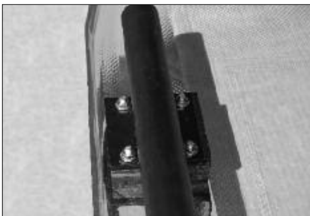
Fig. 22 Crossbrace Assembly
