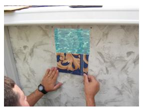
Pull down on flap and tape along the bottom edge.
