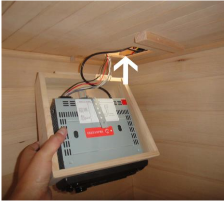
FIG 15.3 Feed the wires up through the roof
