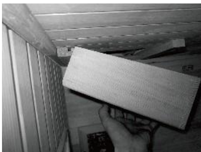
FIG 15.2 Installing the Radio Wood Housing
