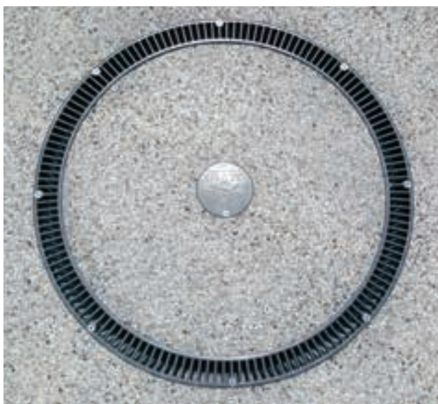
Top view of completed Full Circle® drain
