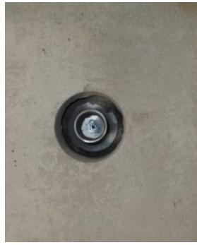
**STEP 3 : Cementing the anchor sleeve in the concrete.**
