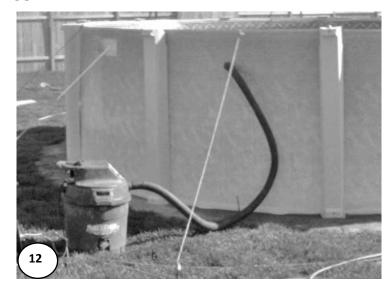
f. Close the skimmer opening with cardboard and adhesive tape so that the suction of air works better. (Image 13)
