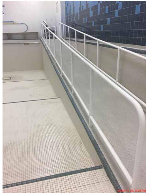
2 RAIL ADA RAMP RAIL CAN ALSO LEVEL OUT TO POST WITH NO P-LOOP
