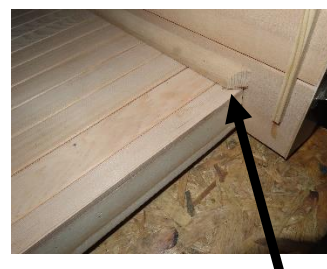
Trim molding of FRONT WALL PANEL resting on the FLOOR PANEL on the interior
