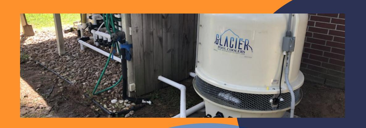
YOUR CHILLER NEEDS FRESH AIR! Do not install your unit in an enclosed room where the unit will suffocate. This is an air cooled system. It needs fresh air in, and a place to exhaust the heat out of the water. Air flows from the bottom and out through the top, thus condensation will appear above when close to a ceiling. For best results, install outdoors or in a very well ventilated area.
