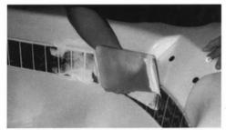
Using a rubber float, spread the silicone grouting into the grout joints of the tile and trim.
