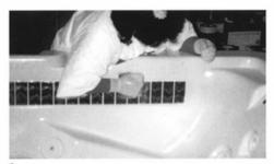
Smooth and clean the grouting and surface, using light strokes to groom the grout and rid the tile surface of excess materials.
