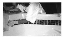
Clean the silicone grout off the tile using a scrubber saturated with one tablespoon of liquid dish soap. The soap serves as a lubricant only.
