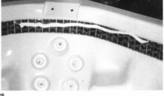
After allowing 30 minutes for the silicone adhesive to dry thoroughly, apply about half a tube of grouting (slow tack) to the tile surface.
