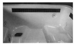
Press the tile firmly into place. The silicone adhesive (fast tack) cures quickly so work with small runs – no more than four or five at a time.
