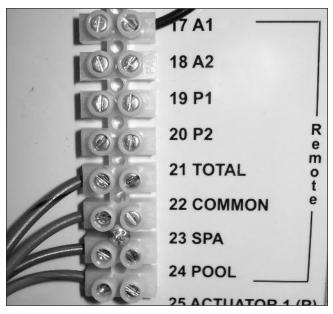
Fig. 10: Heater Wiring Block — Analog Heaters
