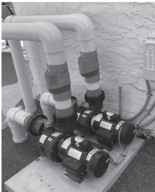
Figure 8 Check Valves Installed
