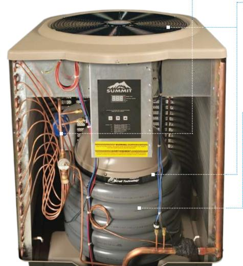
This technology relies on the efficiency of the Scroll compressor, our exclusive soundproofing and the swept-wing fan blade
