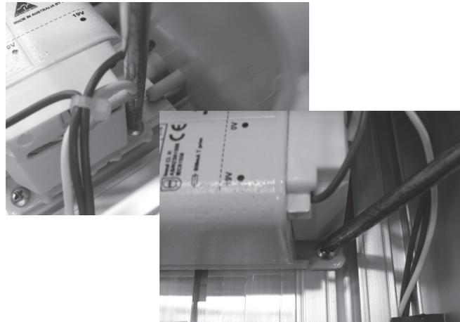
**Step 2** – Place transformer in correct location, replace the rear screw first using a long blade Phillips head screwdriver then the front two screws using a Phillips head screwdriver (two point).
