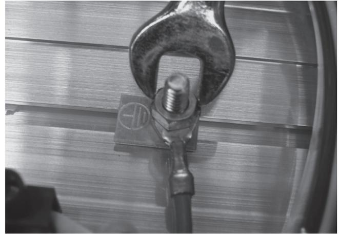
**Step 2** – Reattach the green power cord Earth lead, use an 8mm spanner to tighten nut.
