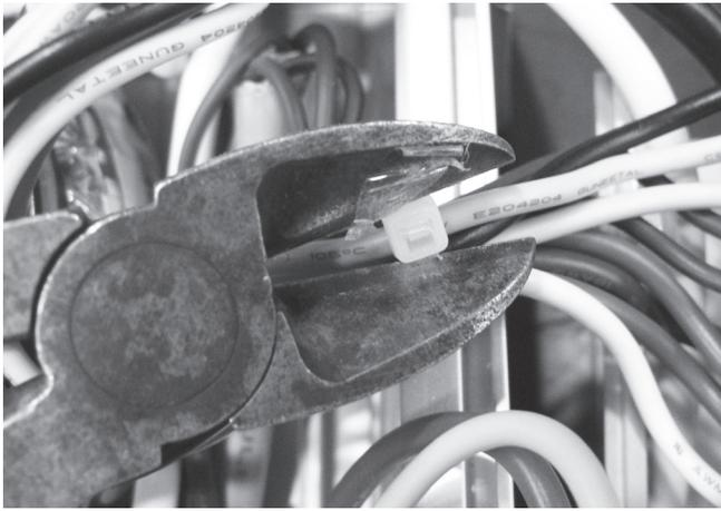
**Step 5** – Remove the appropriate cable ties with a pair of side cutters. Take special care not to cut or damage the wiring.
